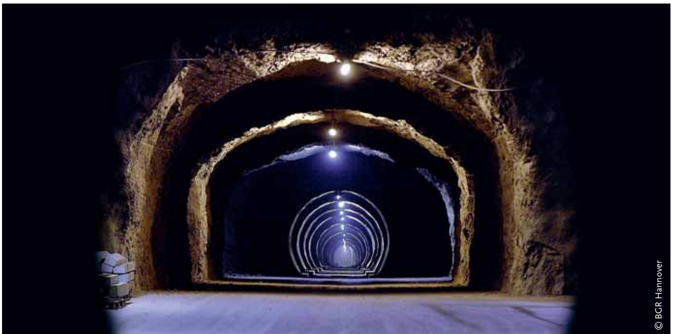
FIGURE 1: Exploration tunnel in the international Mont Terri Rock Laboratory (Switzerland). For about 20 years, scientists carry out experiments on the long-time safety of repositories in Opalinus Clay (sedimentary rock).
